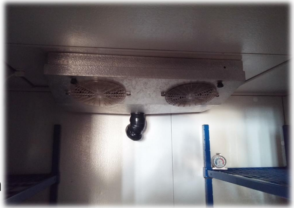
Walk-In Refrigerator at Brinckerhoff Elementary School.
