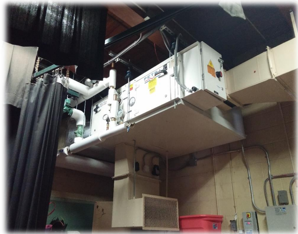
Existing constant air volume system at the Evans Elementary School
